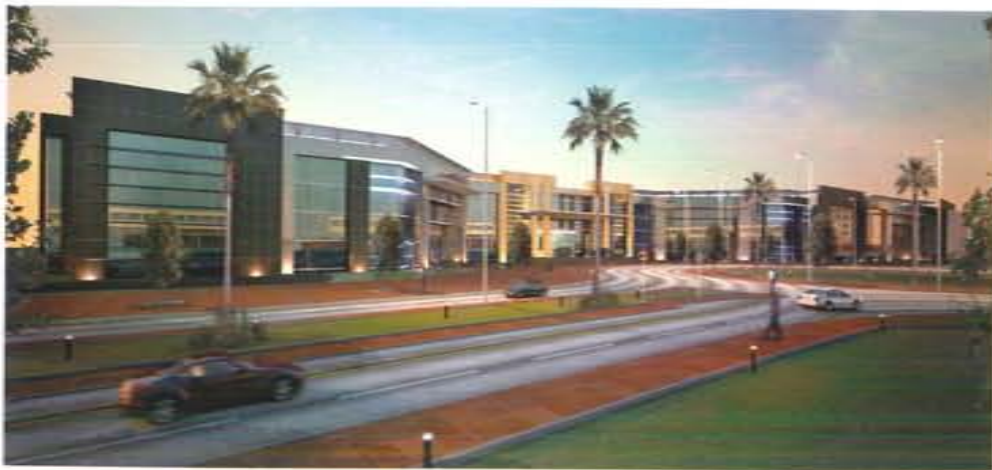
Above: A Mimar-designed commercial and office building located in Dubai Investment Park.
